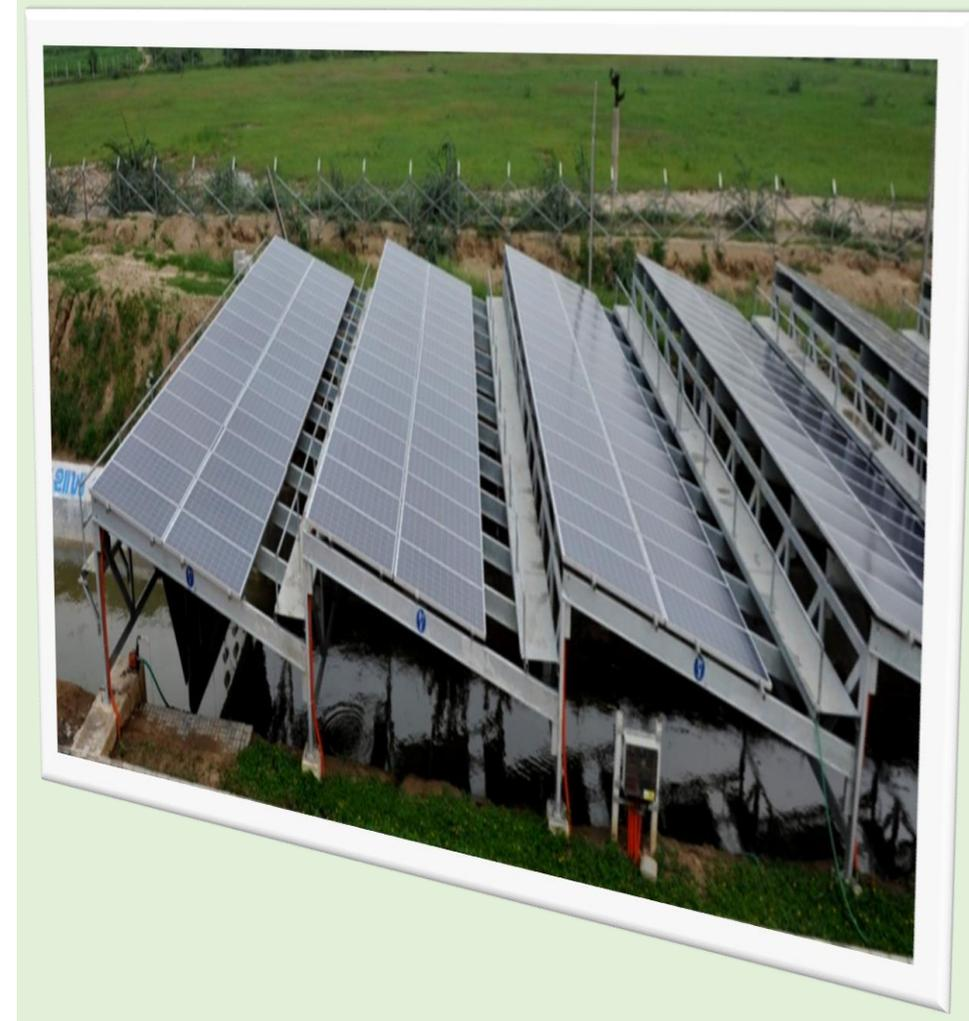
**Installed Capacity****1 MWp****Canal Length used****750 Meters****Nos & Type of Module****Total 3616 Nos / Polycrystalline
