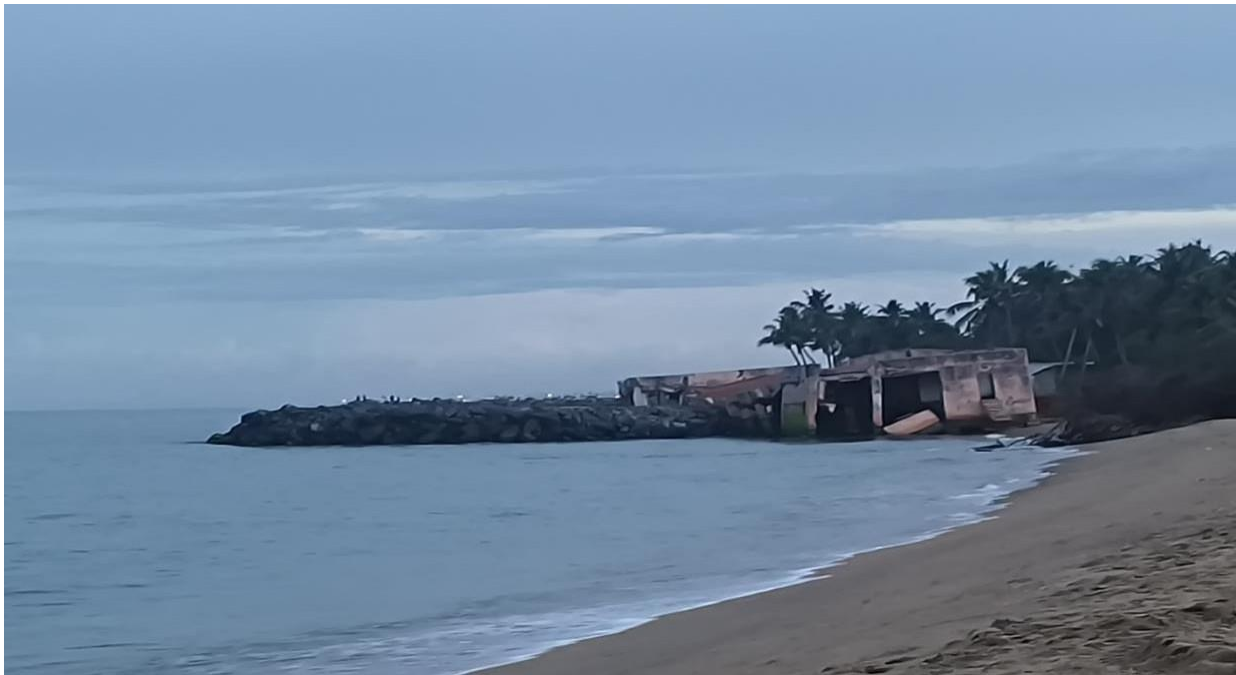
Source: By Author During Field Investigation. Construction of Groynes in Kalapet Beach
