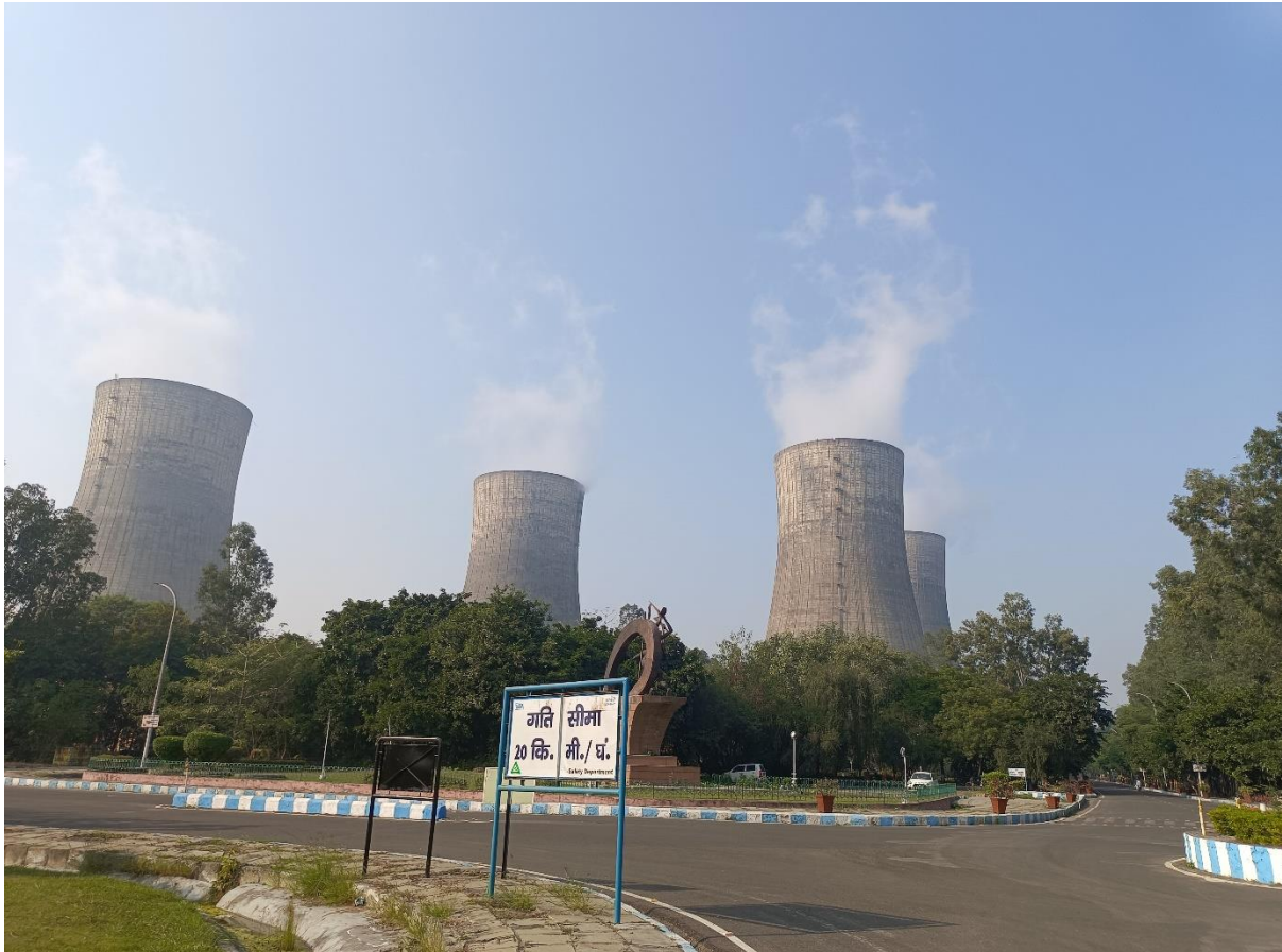
Figure 9.1 Cooling Tower at NTPC Dadri
