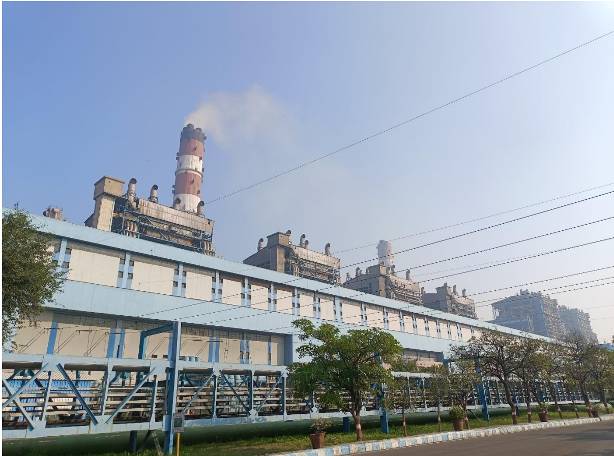
Figure 9.2 Gas Tower at NTPC Dadri
